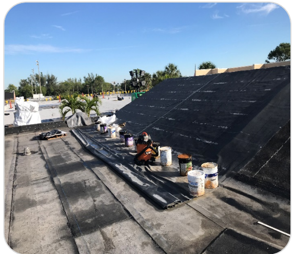
Pitched Roof Before & During Shingle Install
