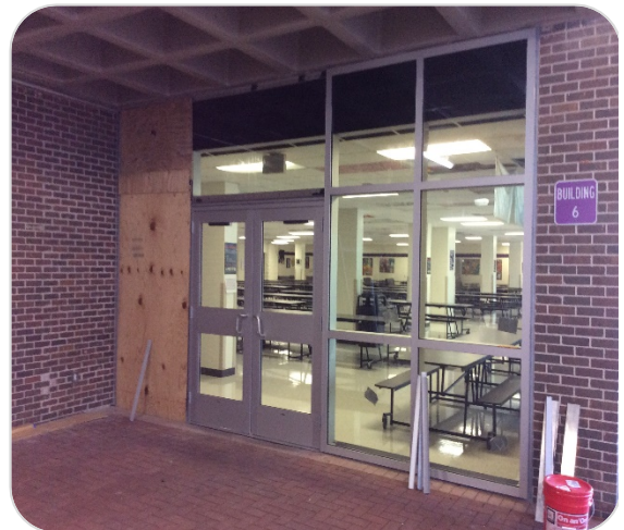
Progress During Window Upgrade Project
