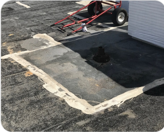
Before Roof Conditions
