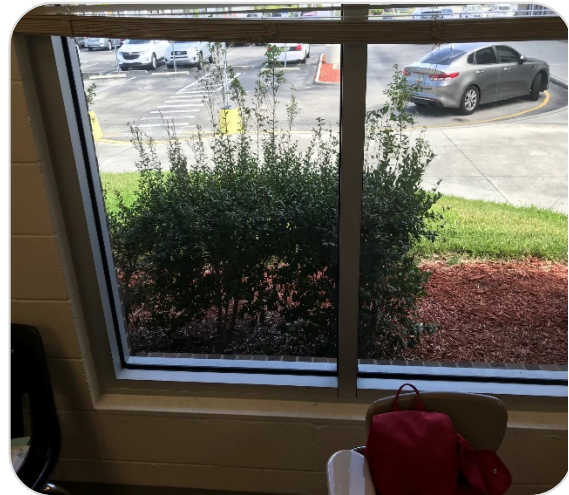
Completed Window Upgrade Project
