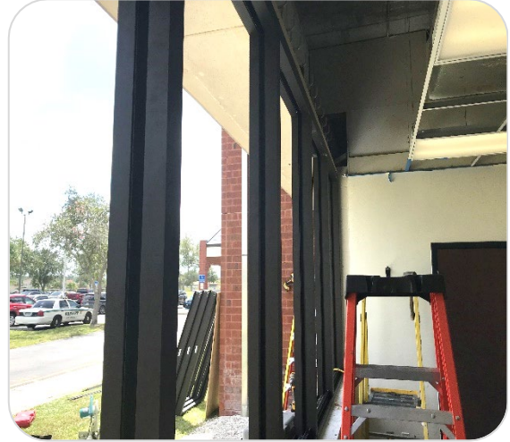
New Window Frame Installed in Front Office
