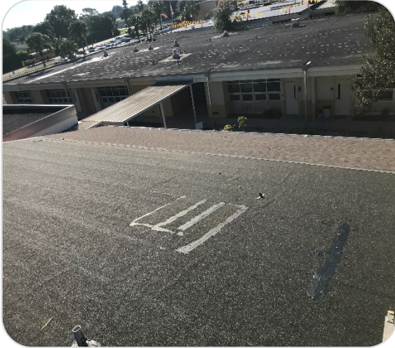
Flat Roof Progress
