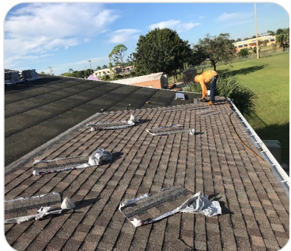
Pitched Roof Before & During Shingle Install
