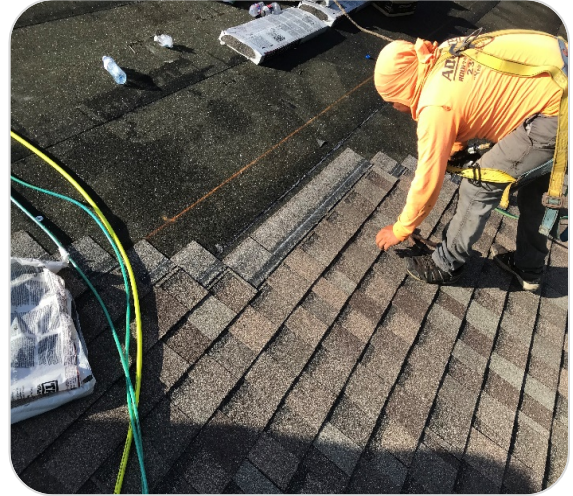
Pitched Roof Before Shingles & During Shingle Install
