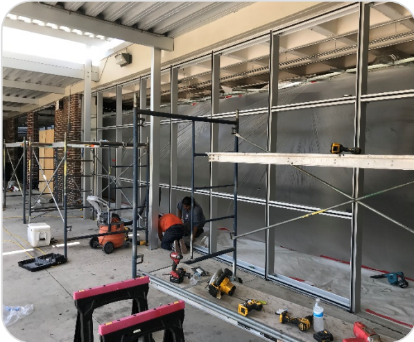
Progress During Window Upgrade Project
