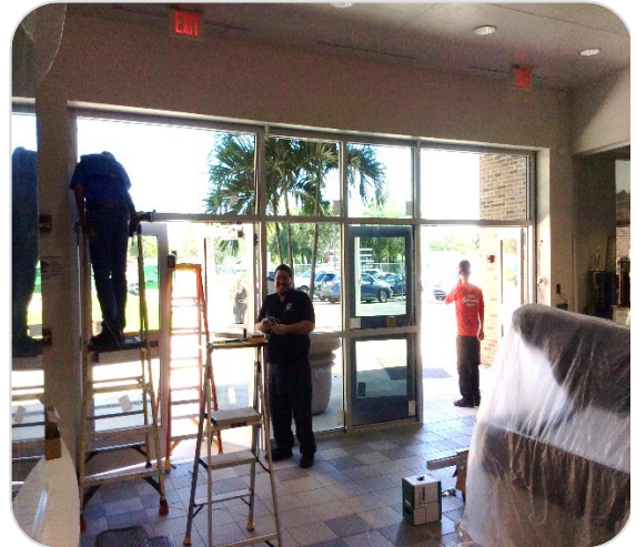
Progress During Window Upgrade Project
