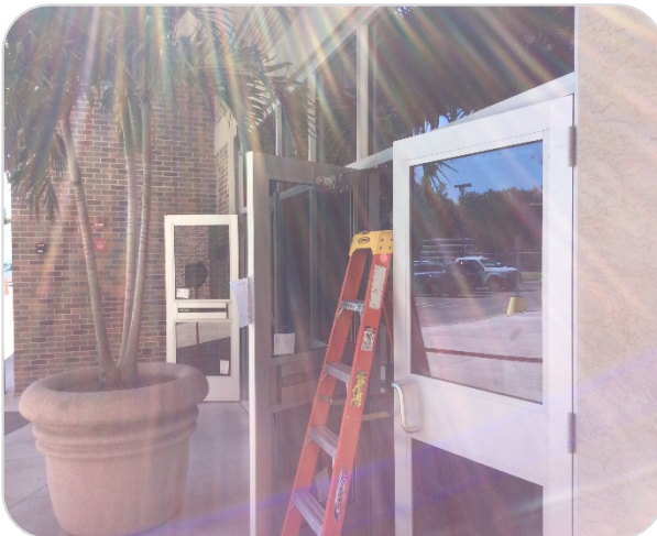
Progress During Window Upgrade Project
