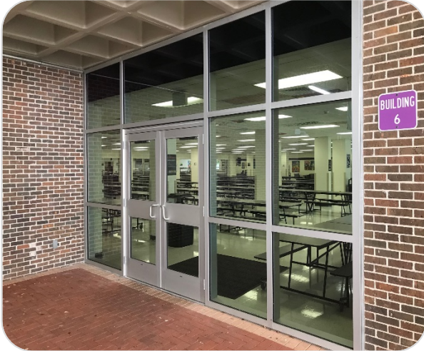
Completed Window Upgrade Project
