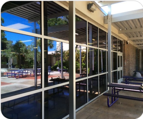
Completed Window Upgrade Project
