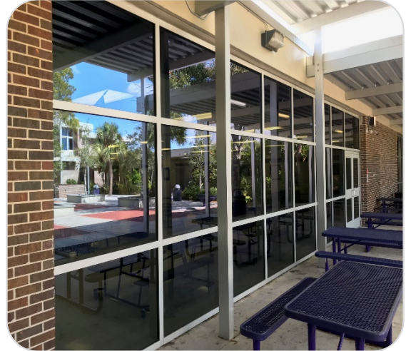
Completed Window Upgrade Project
