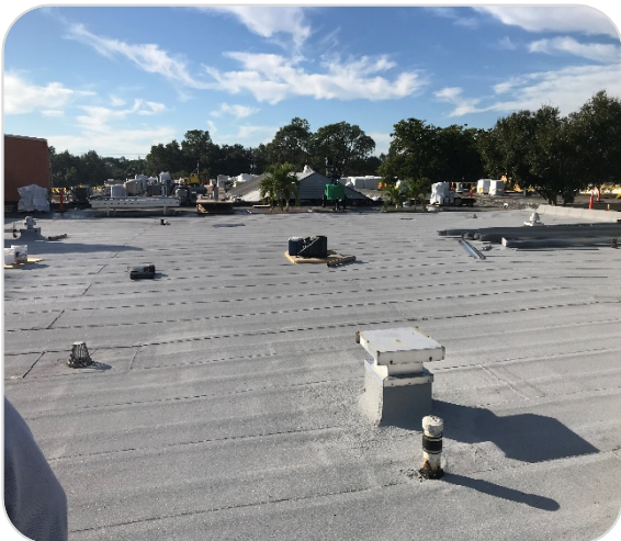
Flat Roof Progress
