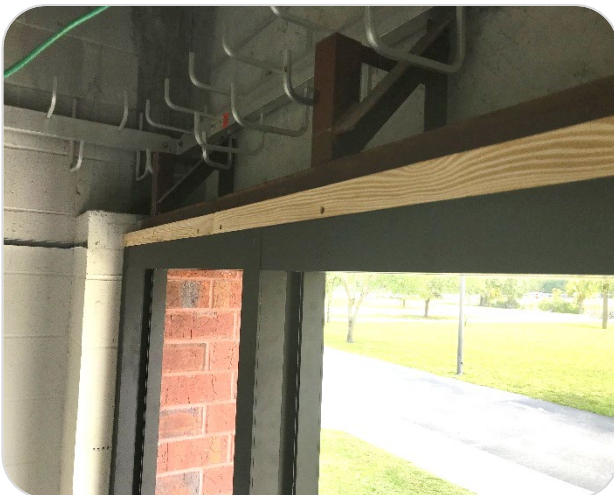
Window Header Reinforcement for Window Upgrade Project
