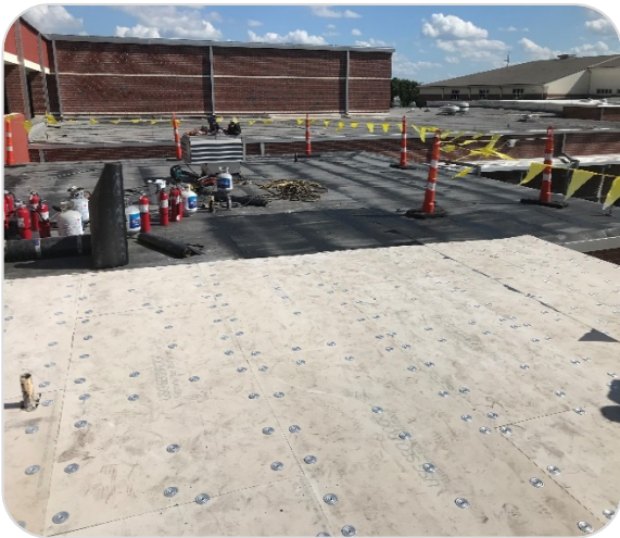
Flat Roof Progress
