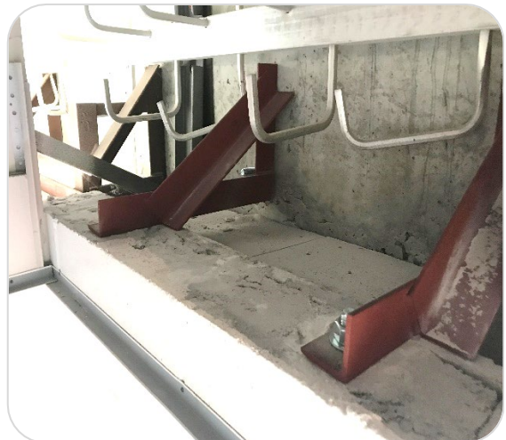
Block Panel Reinforcement for Spandrel Framing for Window Upgrade Project
