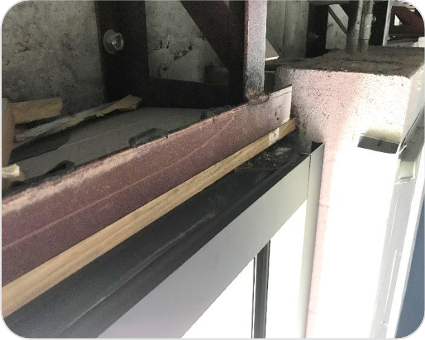
New Window & Header Installation Completed
